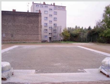
Site: Base course ready for the pitch
