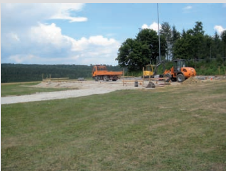
Site: Preparation of the foundations and base course
